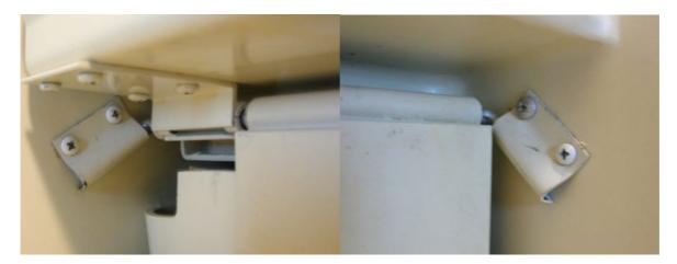
First remove the four screws that hold the fold down shelf and sink. There are 2 located on each side beneath the shelf. Then lift out the shelf and sink.
