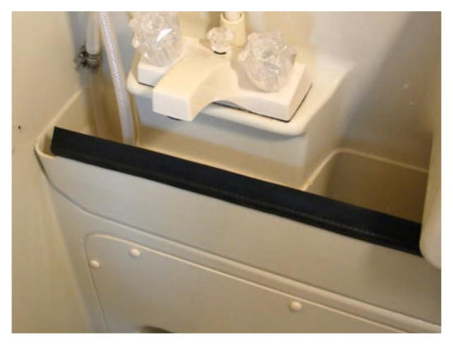
Next I cut the new gasket to length and pushed the U channel down over the plastic edge of the basin. It is a VERY tight fit so some firm pressure is required. THAT'S IT! Now replace the shelf and sink and NO MORE SPILLS FOREVER!
