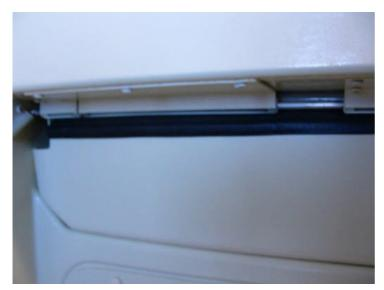
Once you replace the Shelf and sink the gasket will bend behind the hinge and fill the gap between the sink back and the catch basin.
