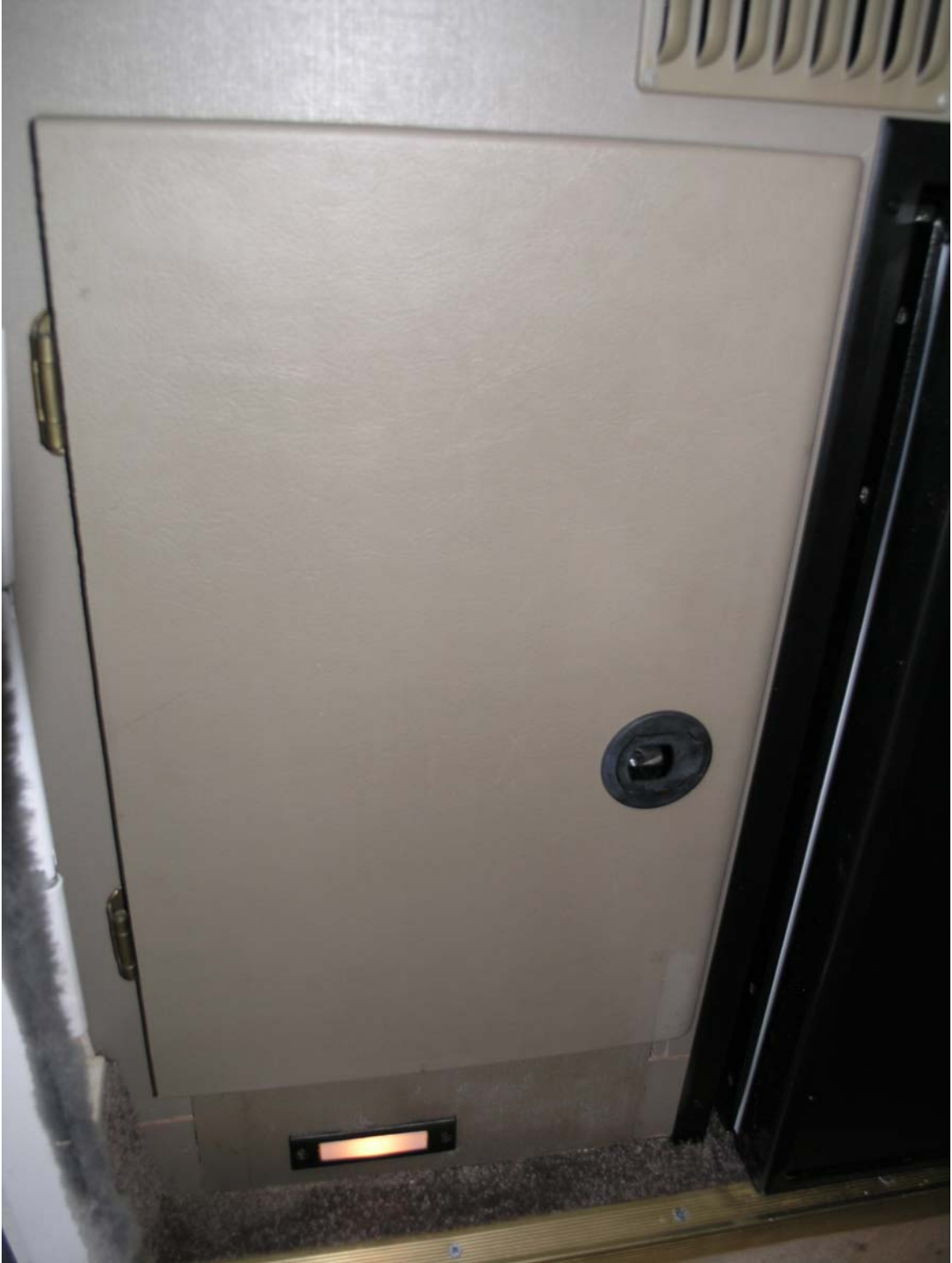
The new door made from the old refrigerator door.
